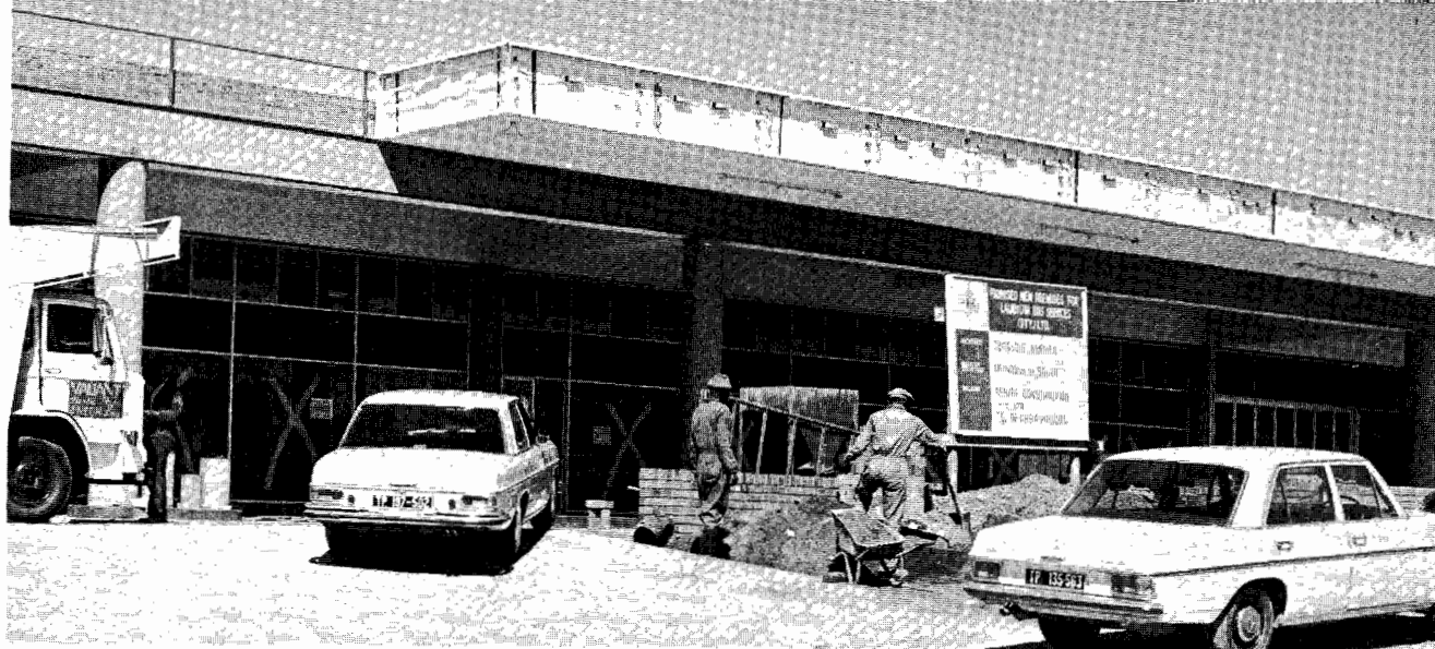
A new garage in the course of construction at Laudium.
